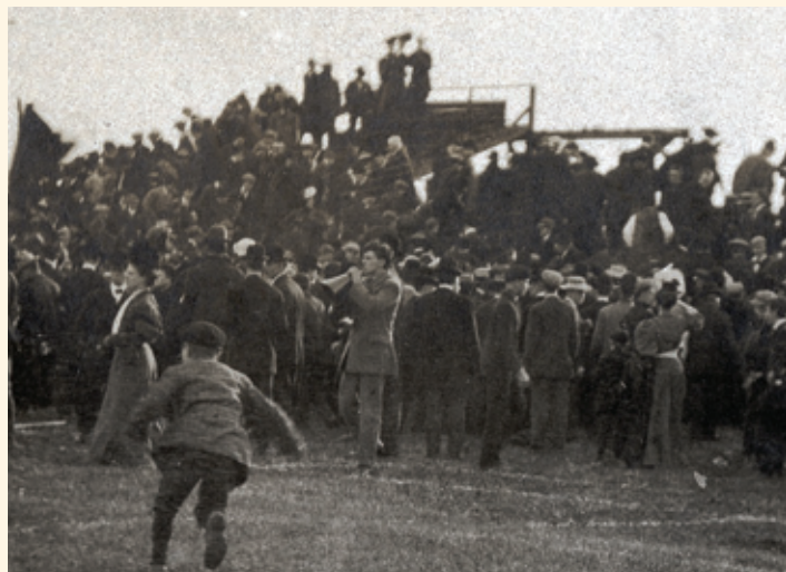
Bleachers Collapse at Star Park, 1906, Photo by Frank A. Math. [Archives Image 11-0943]
